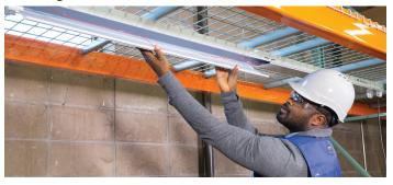
2. Cut the wire leads coming from the sockets and remove the sockets and socket bars on both ends of the fixture.
