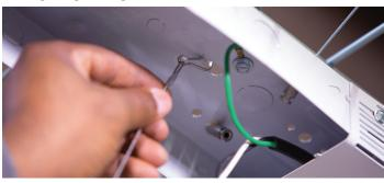
**5.** Make electrical connections for input power (via the included Power Quick Disconnect) and fixture ground. 0-10V connections optional. **For 8' kits only:** connect the LED module wiring between the 2 strip pans via the pre-wired linking connector.
