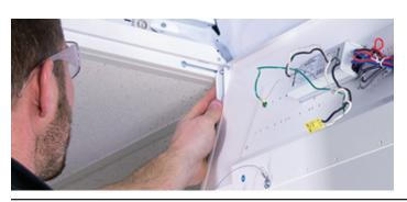
**4.** Insert the doorframe of the retrofit into the keyholes of the support brackets and slide the unit into place.
