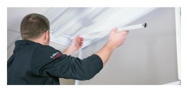
2. Install support brackets (x2) and secure with tek screws.
